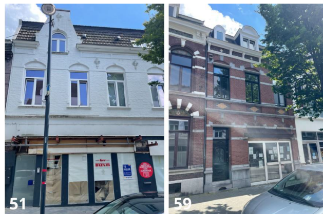
FIGURE 8 - Retail properties with the highest expected residential utility (Krus, 2024)
